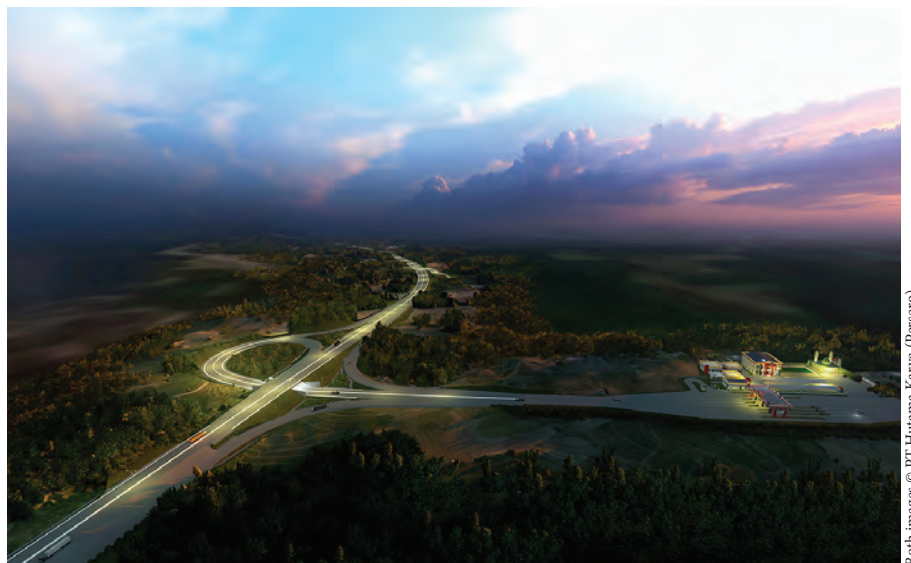
The Serbelawan-Pematangsiantar section of the Trans Sumatera toll road project features 28 km long. Here, PT Hutama Karya also adopted Bentley Systems' digital solutions to improve work efficiency.
