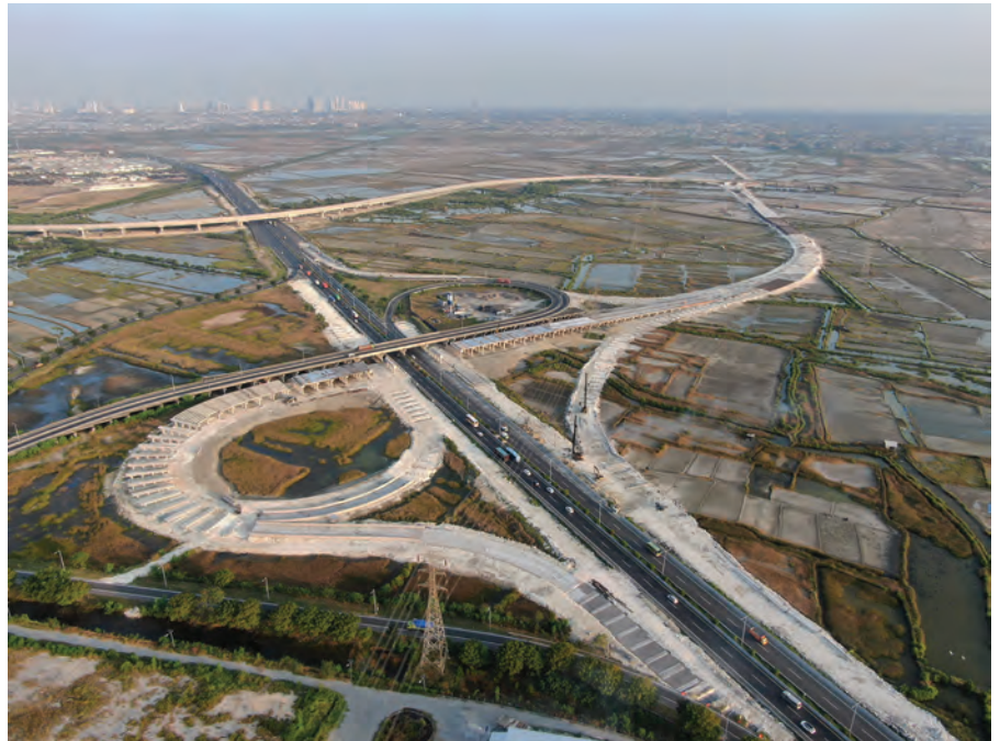
PT Hutama Karya used various digital solutions from Bentley Systems to build the Surabaya-Gresik toll road interchange project in East Java.
