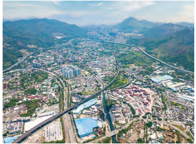
Hong Kong's new Hung Shui Kiu Station will serve the future transport needs of the Hung Shui Kiu/Ha Tsuen New Development Area.
